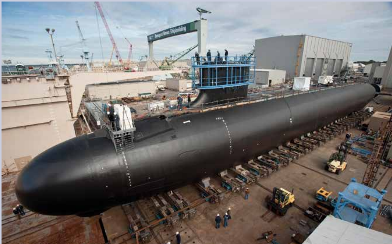
The US Navy has launched a new naval shipbuilding plan that aims to improve the performance of its indigenous shipyards. This photograph shows the Virginia class nuclear-powered attack submarine Minnesota (SSN-783) at Huntington Ingalls Industries' Newport News Shipyard. (©Newport News Shipbuilding)
